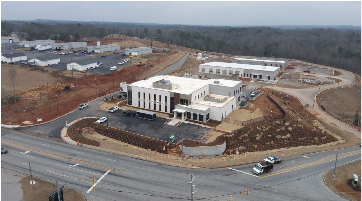
New MetroConnects Headquarters
